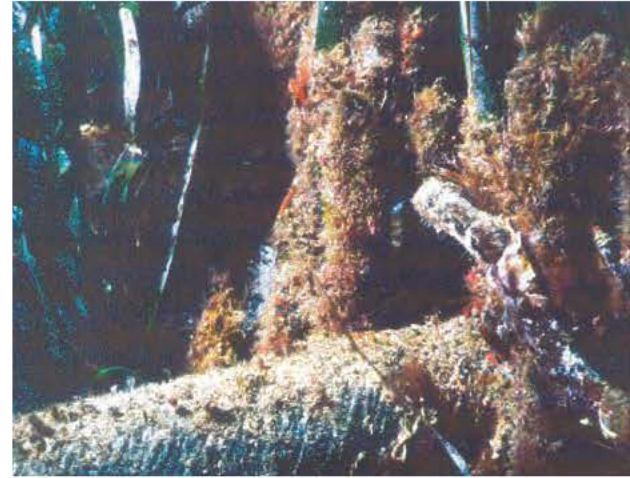
Fig. 118. A cable laid in 1948 between Tour Fondue and Porquerolles (Var, France) is today covered in "matte". The photo was taken on a segment where the Posidonia oceanica meadow is bared, revealing the cable. From Charbonnel et al. , 1995e). Photo by E. Charbonnel.
