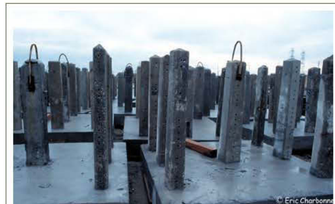
Fig. 89. "Fakir" type anti-trawl protection modules based on reconditioned EDF (Electricité de France) electricity poles. 91 modules of this kind were sunk in 1997 inside and outside the Reserve of Cap-Couronne in the Côte Bleue Marine Park. Photo by E. Charbonnel.
