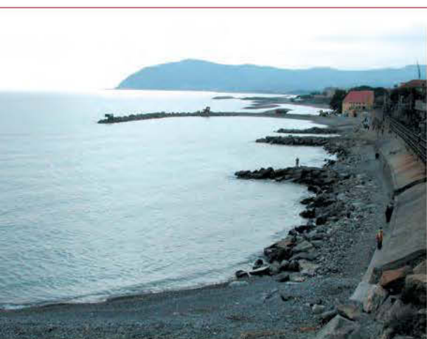
Fig. 63. Cervo (Imperia province) facility for defence against erosion of the coast and the railway line (Settore Ecosistema Costiero archives – Liguria region).
