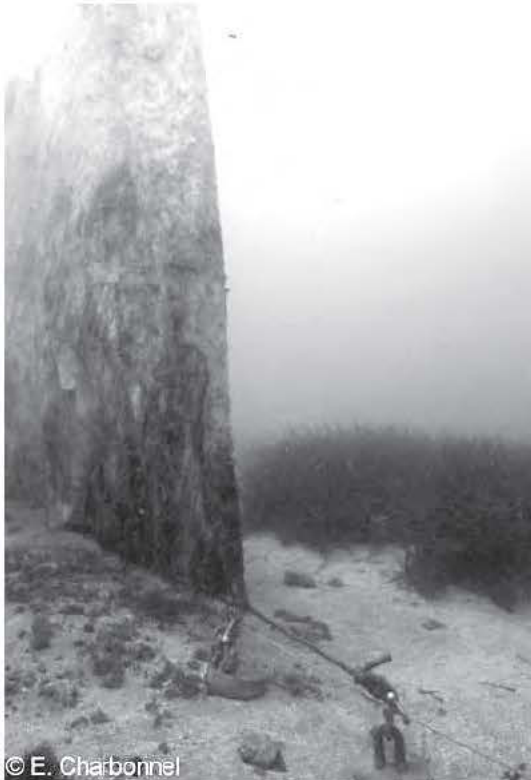
Fig. 73. A geotextile screen (left) protecting a Posidonia oceanica meadow (right) during underwater work on the Canier site (Var, France). Photo by E. Charbonnel.
