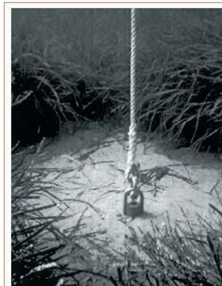
Fig. 81. The fastening ring of a Harmony-type mooring, with the first part of the mooring cable, in a Posidonia oceanica meadow. From Smat Neptune Environnement (2000).
