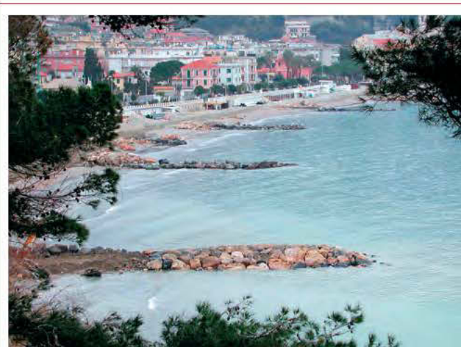
Fig. 66. Laigueglia (Savona province) A facility to defend the coast against erosion (Settore Ecosistema Costiero archives – Liguria region).
