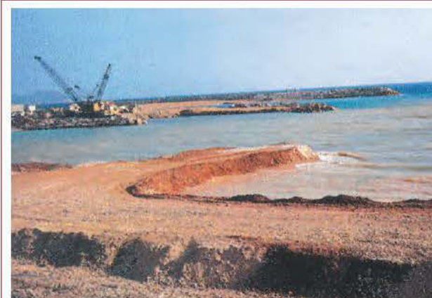
Fig. 59. Developing Le Mourillon's artificial beaches (Toulon, Var, France). Fine sediment is carried off by hydrodynamism. From Astier et al. (1980).
