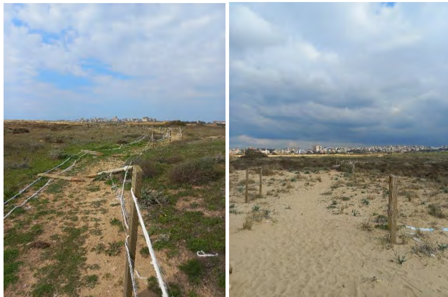
Figure 10. The educational trail and the wooden bridge that need rehabilitation within the Conservation Zone
